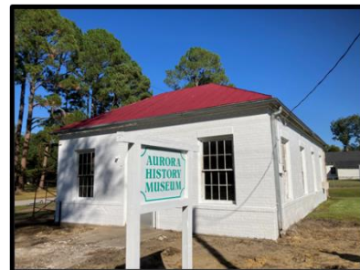
Figure 4.1.2 – Aurora History Museum Renovation
